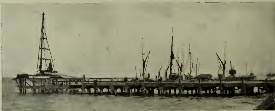
FIG. 5A. TUNNEL CEMENT WORKS, PURFLEET: LOADING JETTY UNDER CONSTRUCTION.
